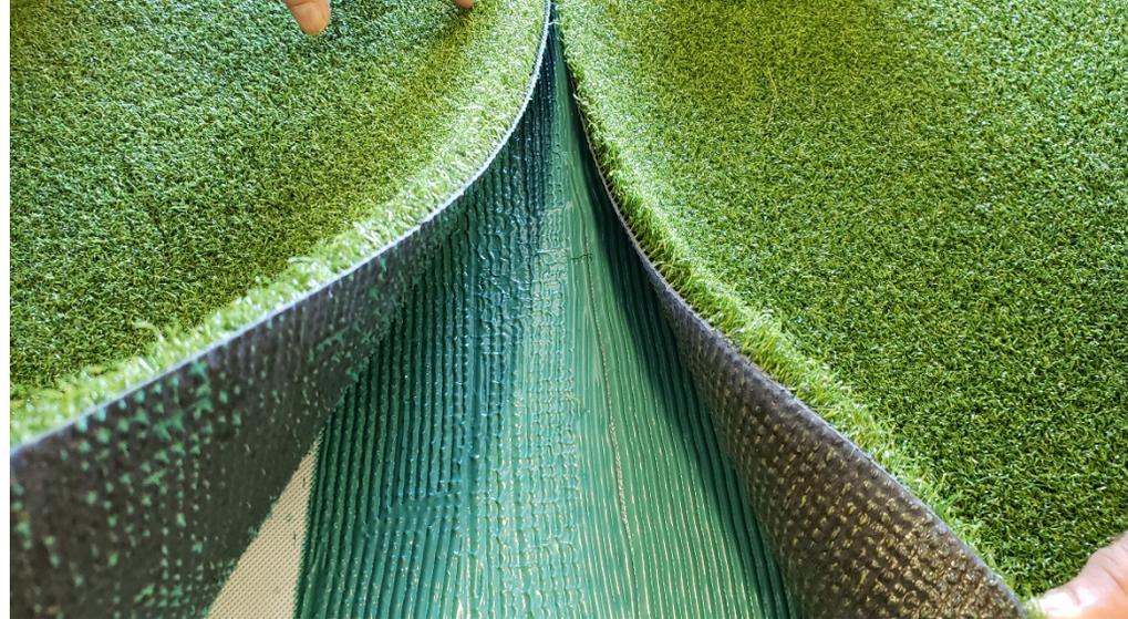
12. Roll seam with a carpet tractor at a 45 degree angle for best results. Rubbing by hand is OK.
