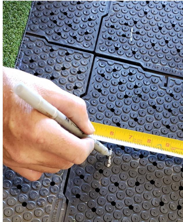
6. Center your seam tape by laying outer edge of tape to six inch marks. Make sure your tape is impermeable. Glue must never stick to the panels.
