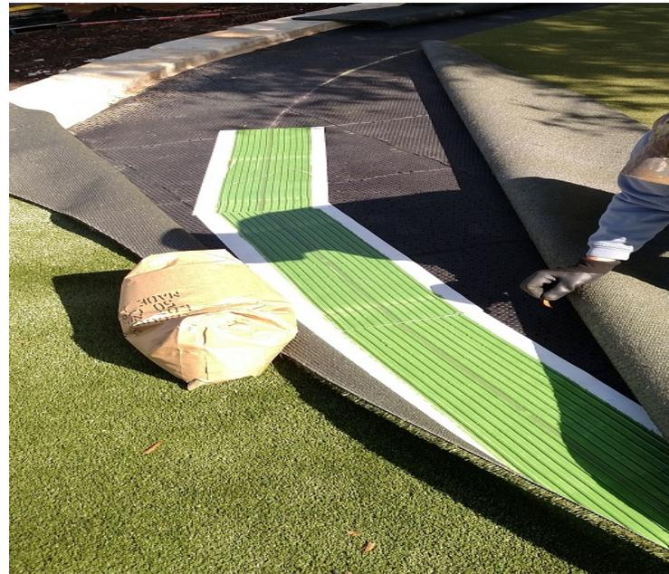
8. If using tubes of Turf Claw MP trim tip of tubes. Do not hold tubes of any adhesive directly over the turf. Having a cloth, pail or cover to work over is important. Glue on synthetic turf needs to be wiped off immediately with a clean cloth. Any glue on turf will be a problem but excessive glue must be removed immediately with a cloth and alcohol or a product like Goof Off. Protecting your turf is essential.
