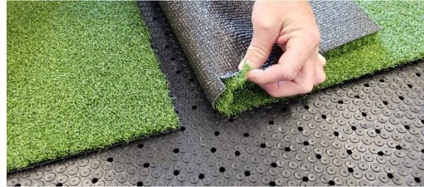
3. Trim/cut turf to fit. For straight cuts you can row cut or you can mark with a chalk line and cut with a straight edge.
