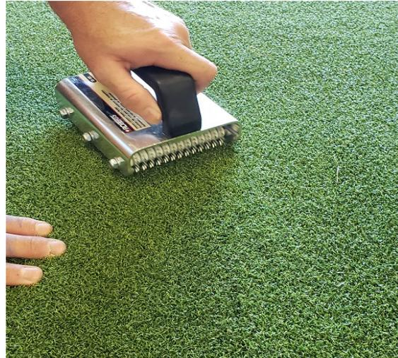
13. If you need to adjust your seam for a final fit now is the time. Turf Claw MP will grab in a few hours and takes 24 hours for a complete cure so you will have time to reposition. Maintain seam contact with weight if you feel there will be any chance of movement from weather or activity near the seam. Maintaining a seam is a critical part of the project.
