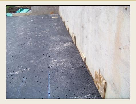
The UBS panels were easily cut with a circular saw in order to achieve proper fit around the walls and outer edges.
